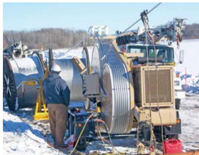
CVI600 Reel Stand can be operated from the AFS404 Puller/Tensioners Control Panel.
