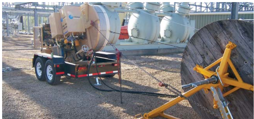
CVI600 Reel Stand can be operated from the FRS404 Tensioners Control Panel.
